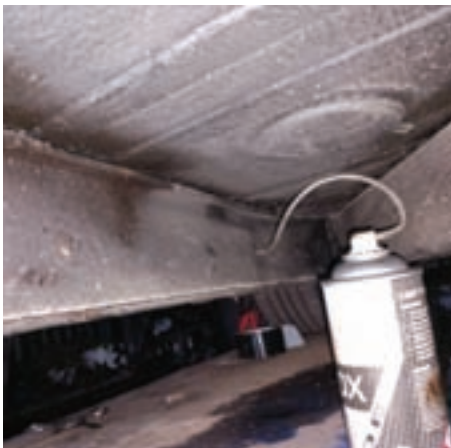
All cavities were injected with anti-corrosion wax.
