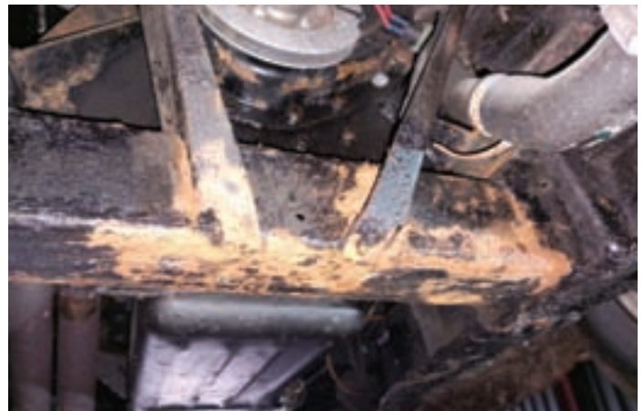
This is the front crossmember after it has been scraped back.
